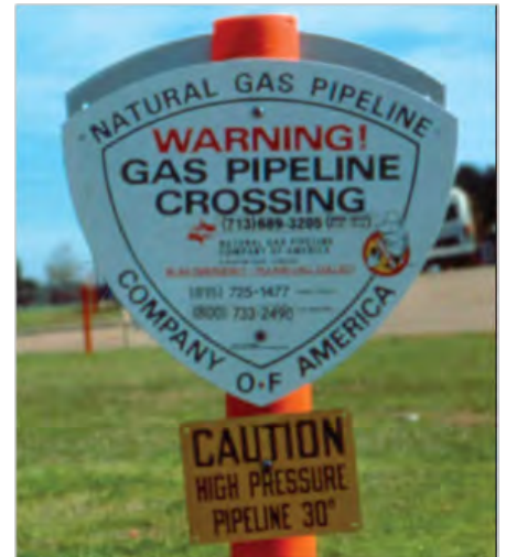
Gas Pipeline Marker
