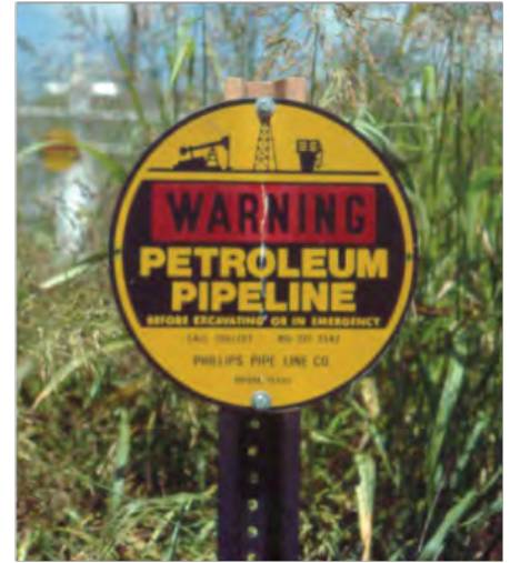
Petroleum Pipeline Marker
